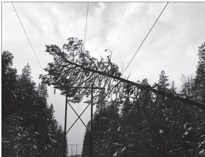
Lineworkers for Klickitat PUD untangled trees from the utility's Glenwood transmission lines after snow and ice in January brought down limbs and whole trees.
